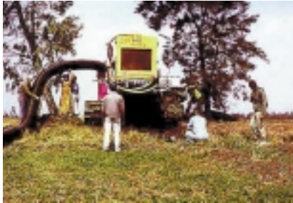
Land drainage installation in Egypt (Photo: DRI)
